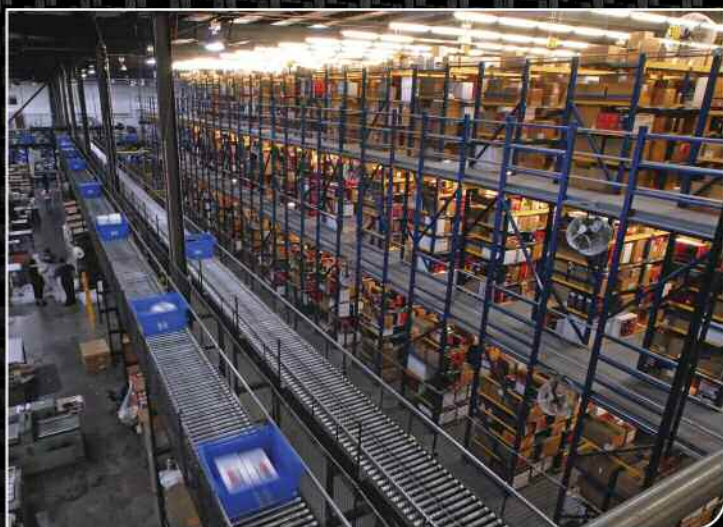
Product warehousing and processing
